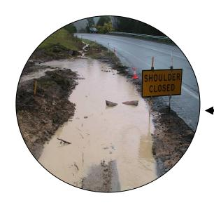
Poor sediment controls at work site allowing soil to wash into waterways.
